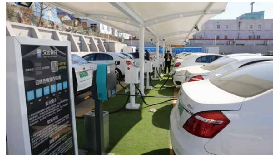
充电集群的建立更为符合当今社会新能源发展的步调。 The clustering of charging piles accord with the development of new energy in today's society.
