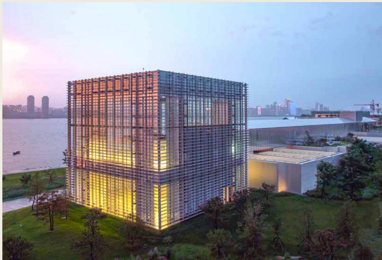
经过多年的筹划、设计、建设，西海美术馆终于揭开神秘面纱，于8月12日正式对公众开放。（图片提供/西海美术馆） After years of planning, design and construction, TAG Art Museum was finally unveiled and officially opened to the public on August 12 th .
